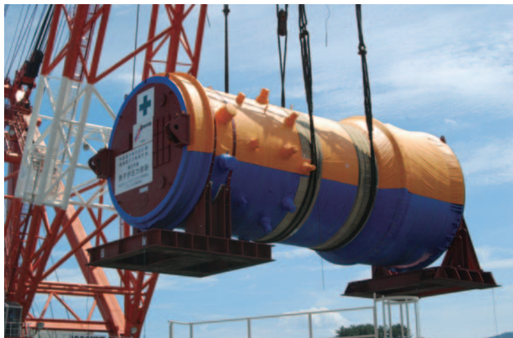
RPV off loaded at construction site
