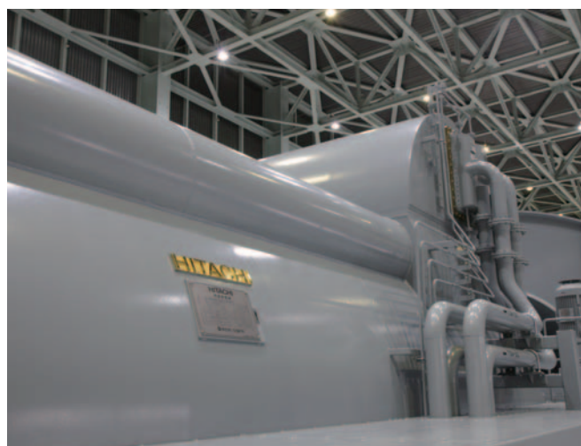
Shimane 3, Nuclear turbine Generator
