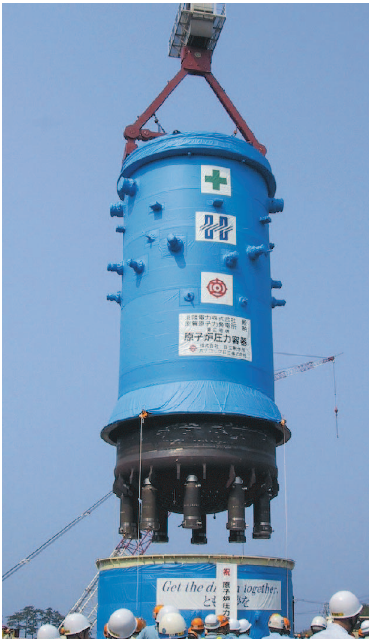
Reactor Pressure Vessel of Shika Power Station Unit No. 2 Being Lifted into Building
