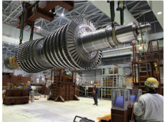
Installation of Turbine
