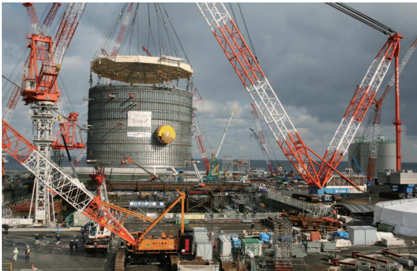
Shimane 3 RCCV Liner module Installation
